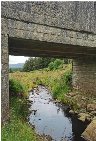
Bridge Crossing No.6
