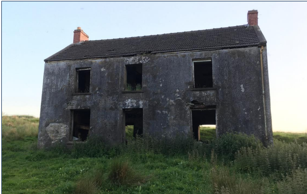
Plate 4-2 Two-storey Derelict Structure with Identified Bat Roost
