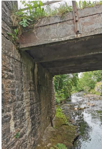
Bridge Crossing No.4 (B)
