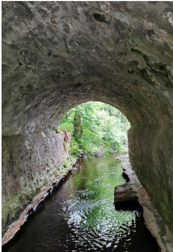
Bridge Crossing No.4 (A)
