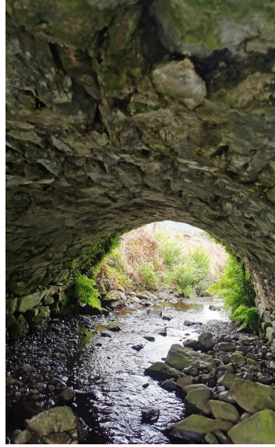
Bridge Crossing No.3
