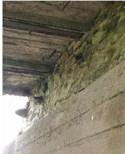
Bridge Crossing No.5
